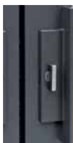
Pull handle on service opening sash
