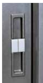
Thumb pull on semi-fixed opening sash
